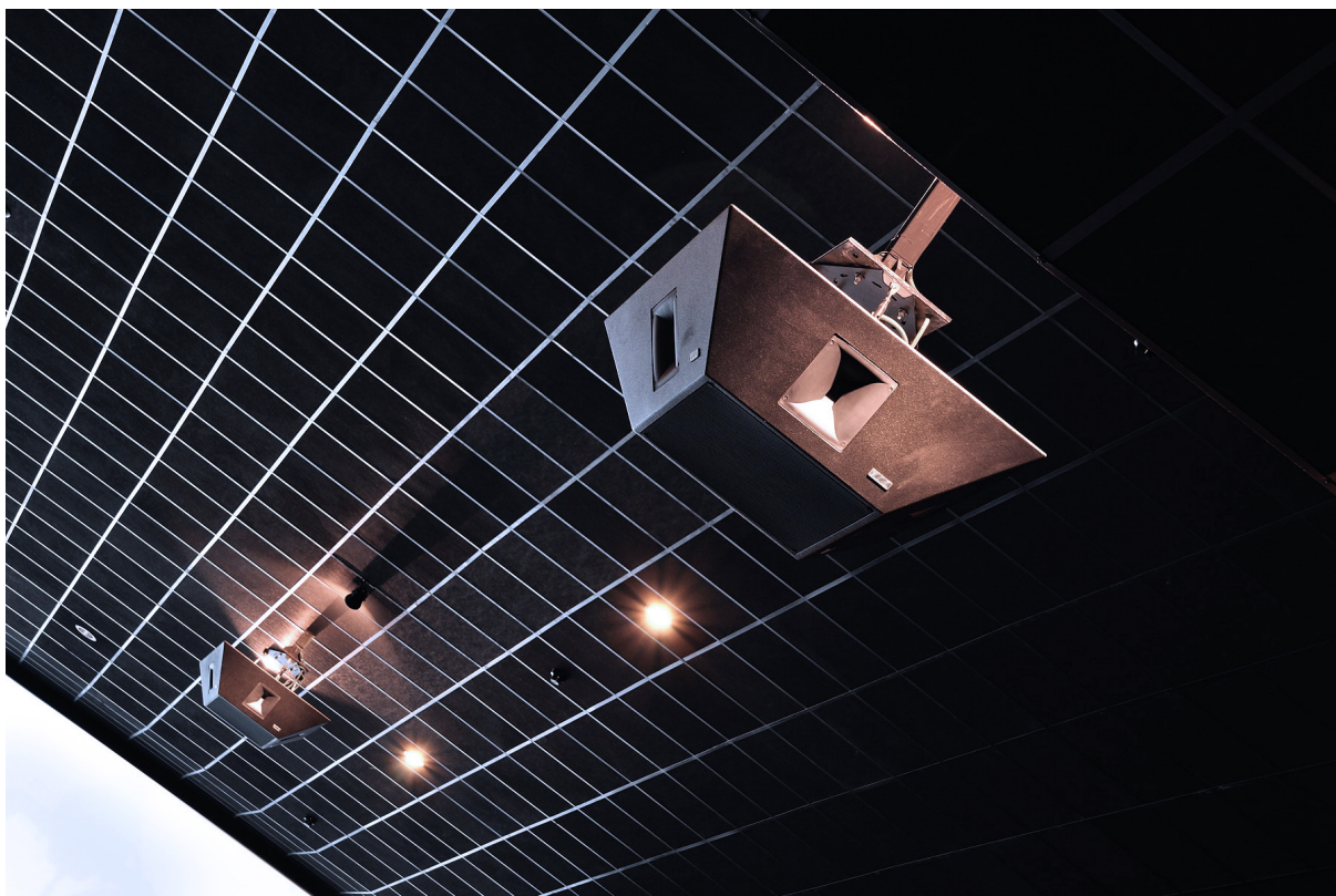
Figure 4: Example of a ceiling loudspeaker solution used in various imm sound theatres around the globe, with wide angular dispersion, light weight, and easy mounting.
